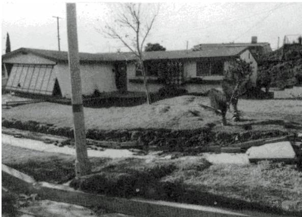
Large fissures in the ground, massive ground movement or slope displacement. Condition: **AREA UNSAFE**
