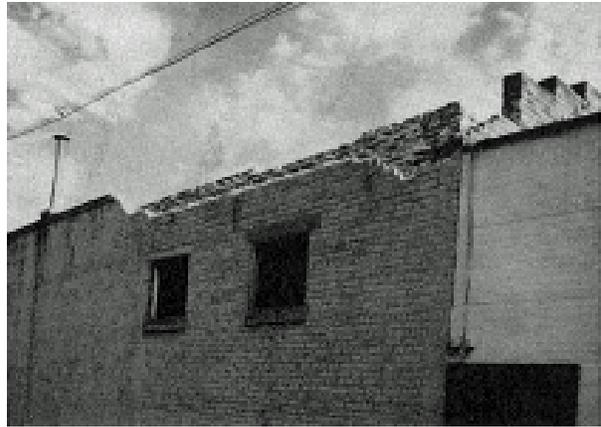
Obvious parapet or other falling hazard. Condition: **AREA UNSAFE**
