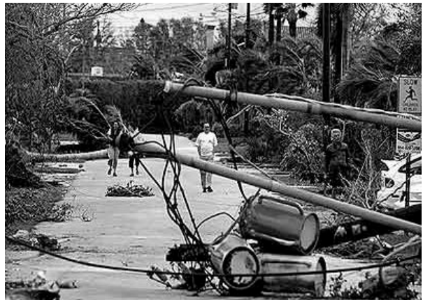
Other hazard(s) present (e.g. toxic spill, ruptured gas line, downed powerline, overturned propane tank). Condition: AREA UNSAFE
